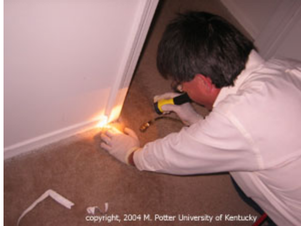
Inspections and treatments must be very thorough
